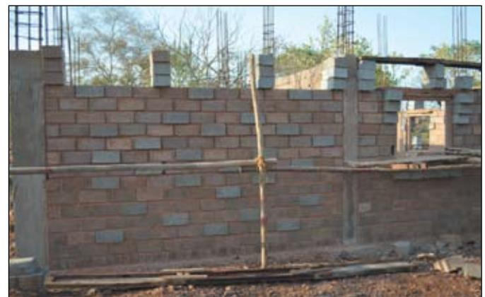
Figure 7. Construction of two-storey house using LC3 blends in progress
